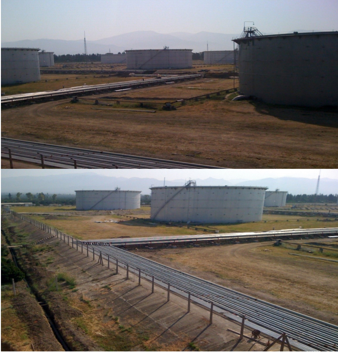
BOTAŞ FILLING FACILITY TANK AREA GENERAL VIEW
