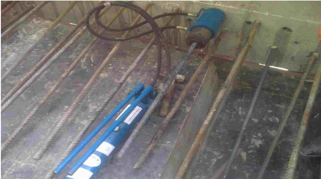
STEEL MANUFACTURING INSTALLATION WORKS
